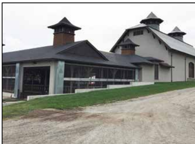
Recent facility upgrades at High Lawn Farm in Lenox, Mass., include a new climate controlled cow barn, above, with Lely robots, alley scraper, waterbeds and push up feeder. The All-Jersey distributor also built a new milk processing plant and sells High Lawn Farm products wholesale across New England.
